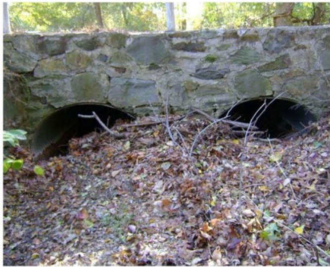
Yard waste can clog culverts and cause flooding. It also brings too many nutrients to the stream, causing oxygen shortages.
